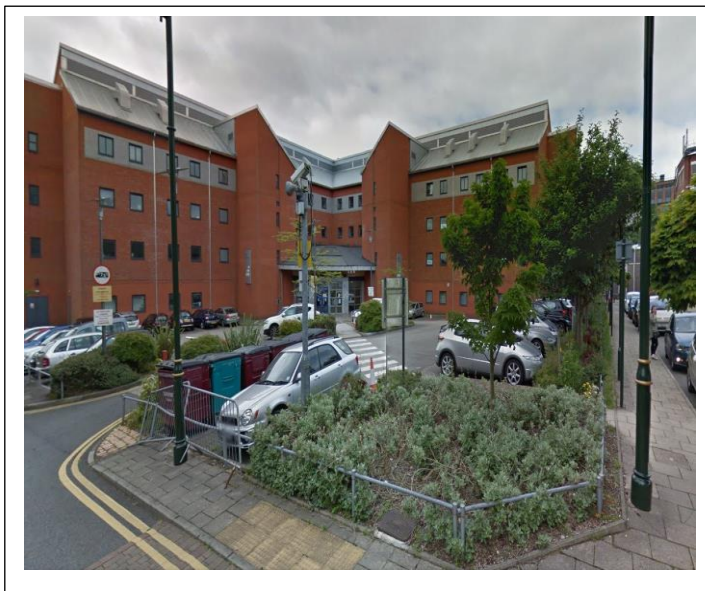
View of Access Road and Car park
